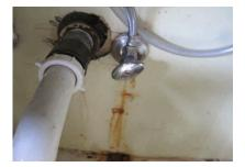
Faucet Functional Components and Conditions The sink faucet is functional. Trap and Drain Functional Components and Conditions The trap and drain are functional. Garbage Disposal Components and Conditions Needing Service Electrical conduit is missing on the garbage disposal wiring.
